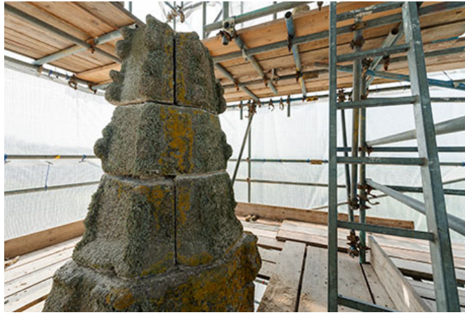
The carefully reconstructed tower pinnacle - St Odolph © Richard Downer
